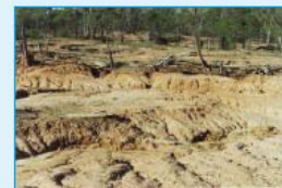
▲ Extreme rill erosion of sodic soils near the Texas-Keytah Bridge.
