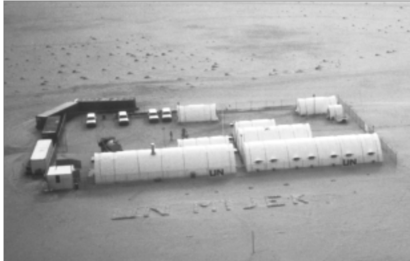
Mijek, Western Sahara. August 1992. Aerial view of the United Nations (UN) Teamsite, the words UN Mijek can be seen spelt out on the ground. The sites are Weather-Haven camps, consisting of white plastic drawn over a steel frame with a prefabricated wood and linoleum floor. On the left are the containers which these sites came in, used as windbreaks. In the top centre and top right are store huts. The smallest of these (top right) is the office for the logistician. The two large white buildings in the foreground house the recreation area, kitchen and pantry (left) and the accommodation, broken down into individual rooms (right). The row of white buildings behind these are the showers and laundry (left) and more accommodation (right). The third, smallest, building behind the accommodation buildings on the right is the operations room where the radio room and the commanding officer's office is located. The silver shed (front left hand corner) houses two generators to power the camp.
